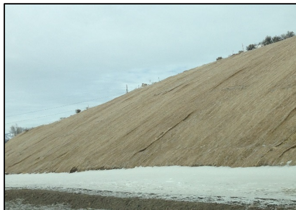
Figure 126. Jute matting applied over a steep slope in Jackson Hole, Wyoming.
