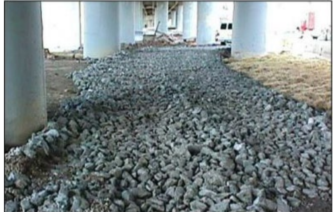
Figure 108. Temporary construction access road (ITD 2014).
