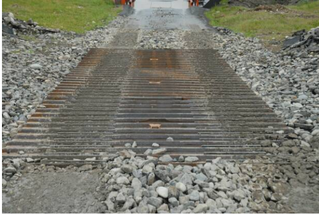
Figure 107. Rattle plates in construction entrance ( The Bag Lady ).
