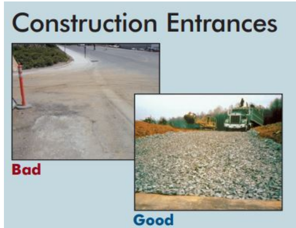
Figure 102. Stabilized gravel construction entrance examples (EPA 2003).
