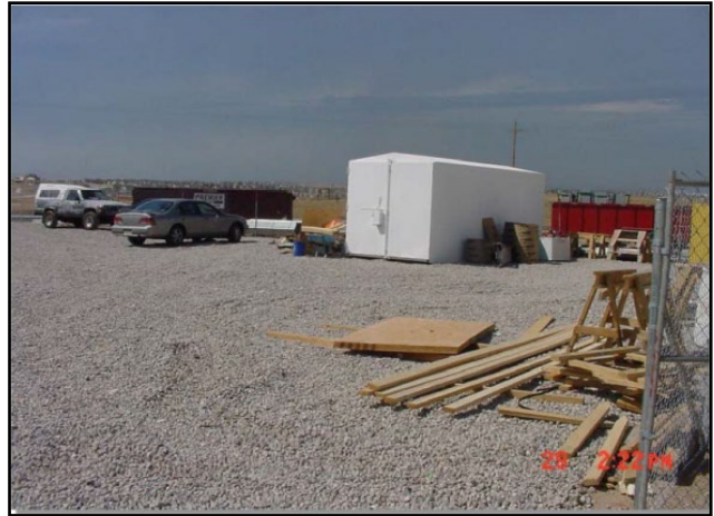
Figure 98. Construction staging area (Colorado UDFCD 2010).
