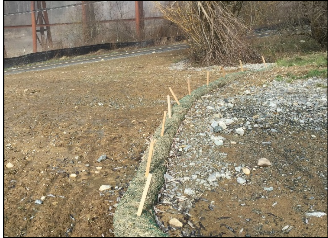
Figure 154. Fiber rolls placed along the top of slope in Sandpoint, Idaho.
