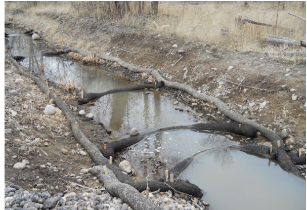
Figure 152. Compost filter socks used to slow and filter runoff.
