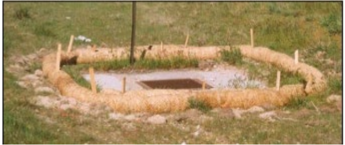
Figure 182. Inlet protection wattle (ITD 2014).
