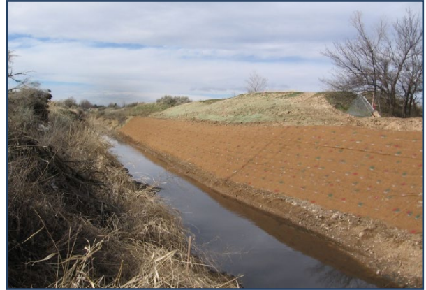
Figure 123. Geotextile channel lining (ITD 2014).
