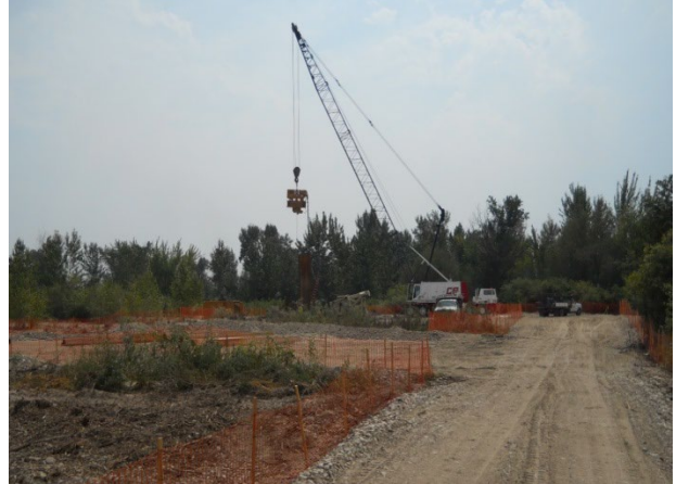
Figure 100. Construction fencing used to define clearing limits on a construction site.
