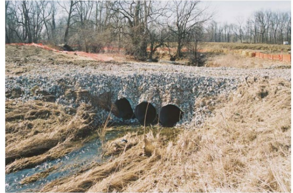
Figure 149. Temporary stream crossing using culverts (Ohio EPA 2014).
