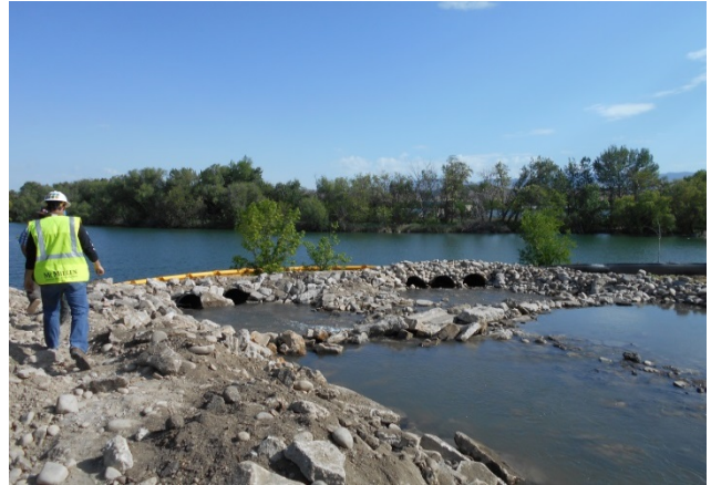
Figure 143. A rock check dam reduces runoff velocity.
