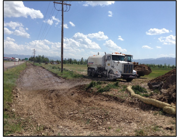
Figure 113. Sprinkling water for dust control on a pathway construction project, Driggs, Idaho.
