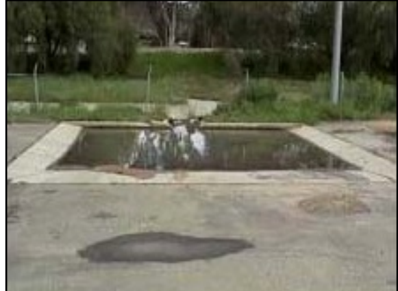
Figure 117. Vehicle and equipment wash area (CALTRANS 2003).
