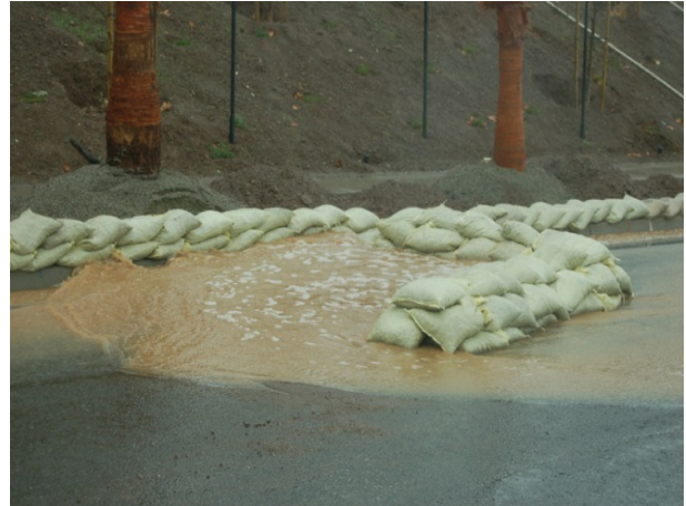
Figure 171. Gravel bag berm ( Natural Building Blog ).
