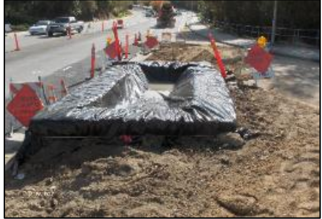
Figure 119. Hay bale temporary washout pit ( On Site Washout ).
