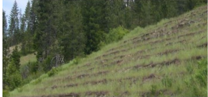
Figure 140. Terraces incorporated into the grading plan (ITD 2014).
