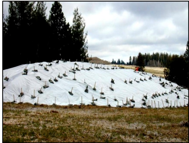
Figure 114. Covered stockpile (ITD 2014).
