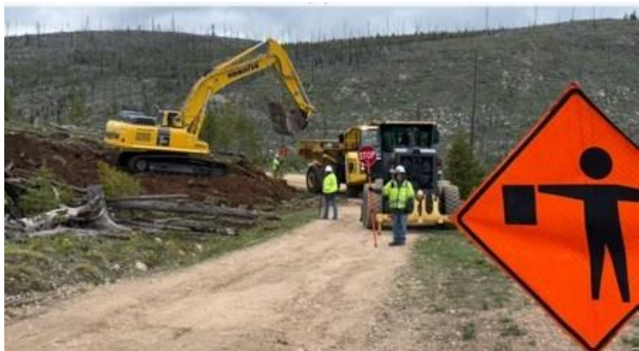
Perpetua crews begin construction of Burntlog Route, May 30, 2026
