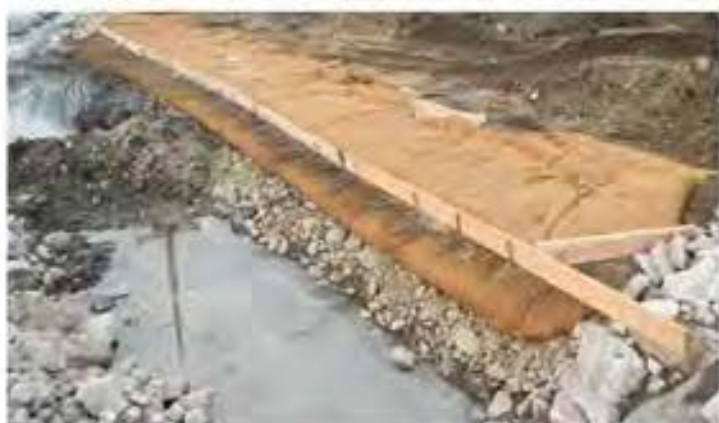
EXAMPLE: FESL INSTALLATION IN FALL DURING DORMANT SEASON
