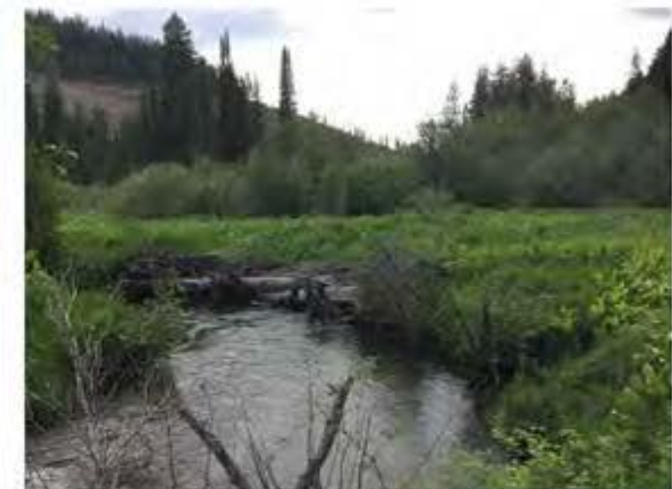
EXAMPLE: INSTALLED TIGHT RADIUS JAM STRUCTURE
