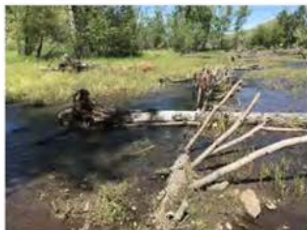
EXAMPLE: INSTALLED LOG FLOODPLAIN ROUGHNESS STRUCTURE
