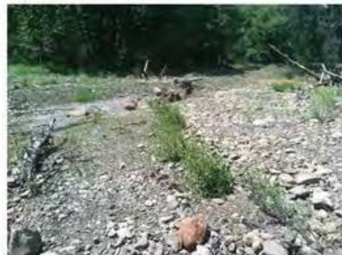
EXAMPLE: INSTALLED LIVE WILLOW TRENCH
