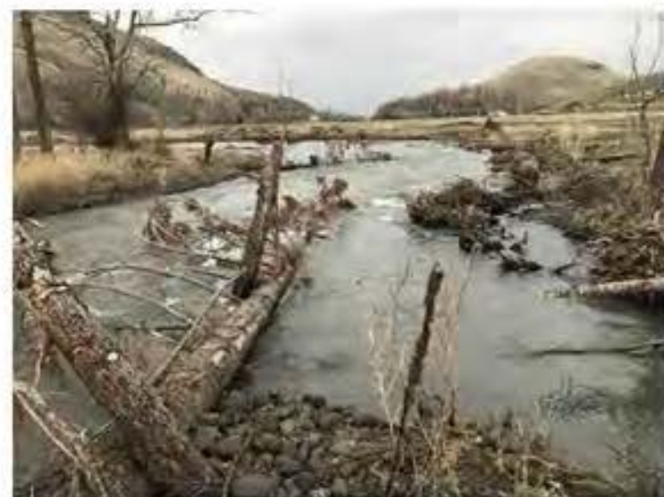
EXAMPLE: INSTALLED TYPICAL SWEEPER LOG STRUCTURE
