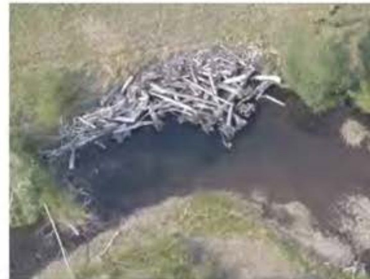
EXAMPLE: INSTALLED BEND JAM STRUCTURE
