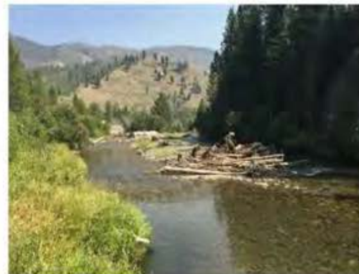
EXAMPLE: INSTALLED APEX LOG STRUCTURE
