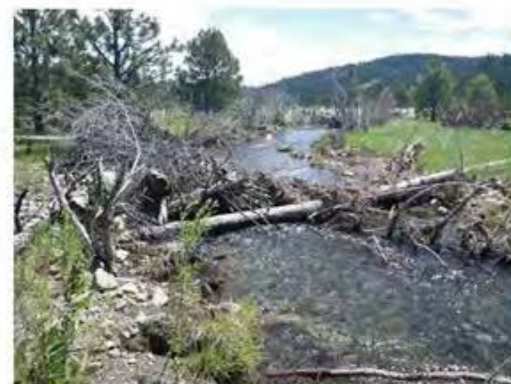
EXAMPLE: INSTALLED CHANNEL SPANNING JAM STRUCTURE
