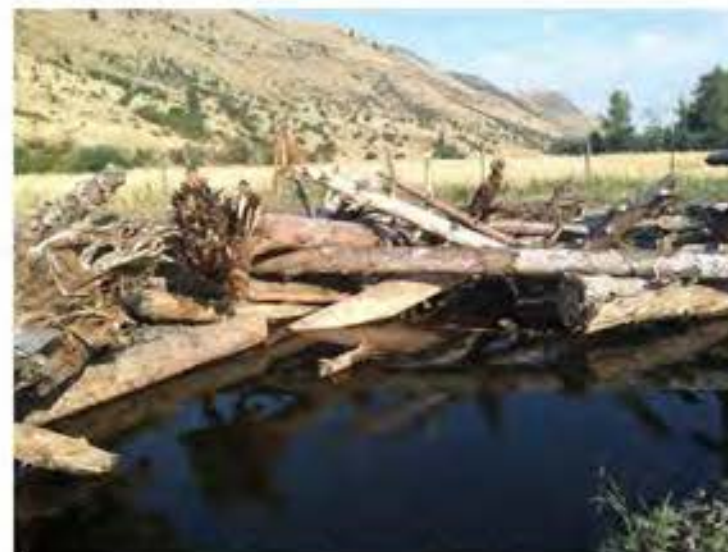
EXAMPLE: INSTALLED TIGHT RADIUS JAM STRUCTURE
