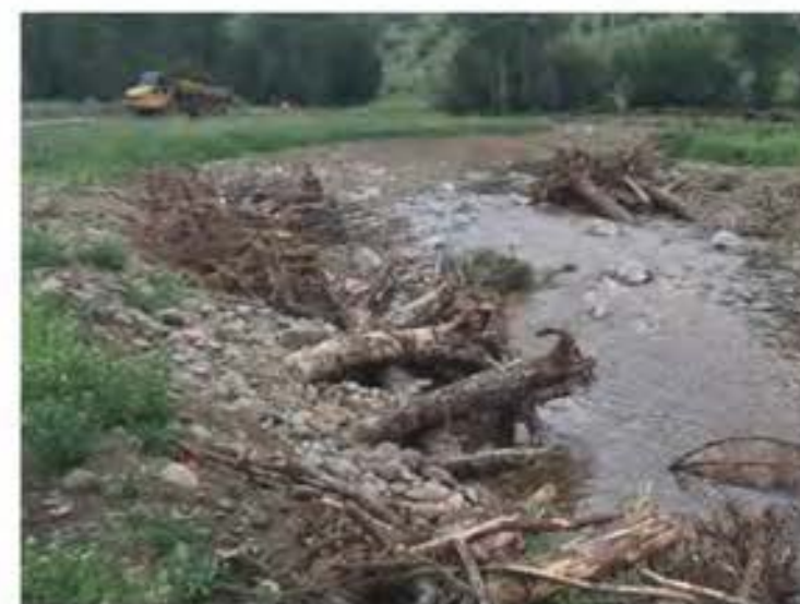
EXAMPLE: INSTALLED TOE LOG STRUCTURE (FOREGROUND)
