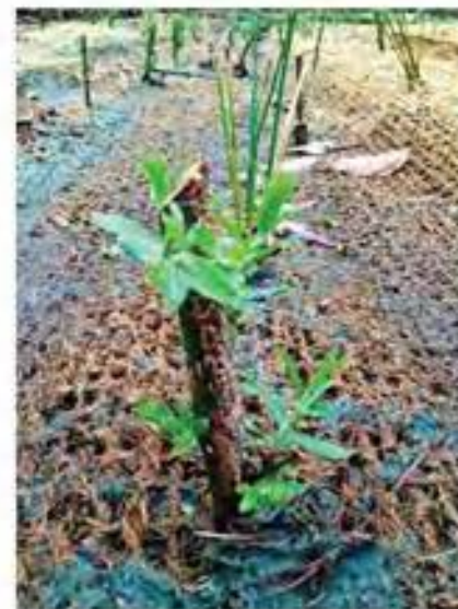
EXAMPLE: INSTALLED LIVE WILLOW STAKE
