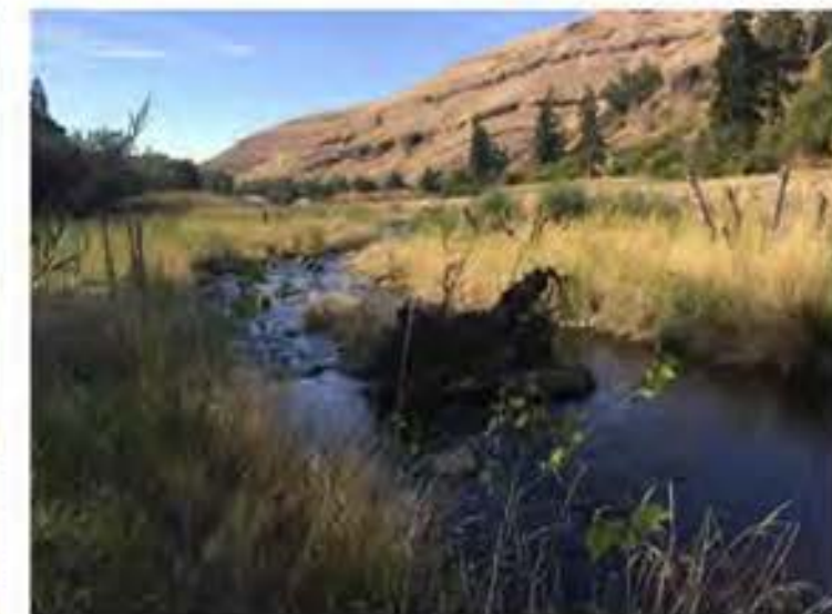
EXAMPLE: INSTALLED SINGLE LOG APEX STRUCTURE
