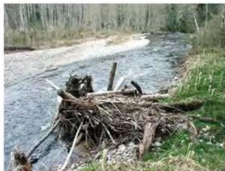
EXAMPLE: INSTALLED TOE LOG STRUCTURE
