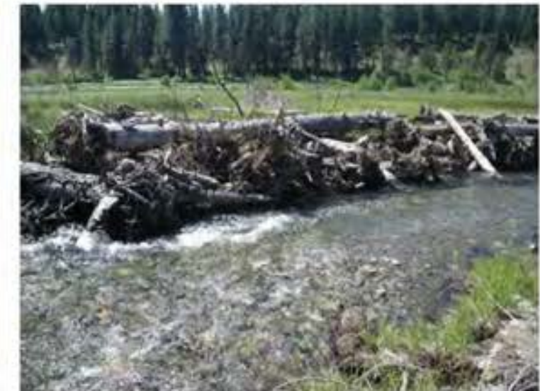
EXAMPLE: INSTALLED BEND JAM STRUCTURE
