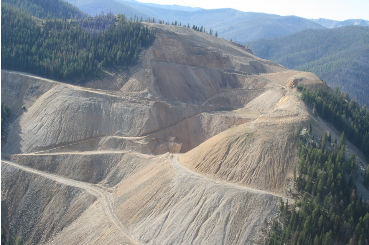
Photograph 6-4: West End Pit showing Partial Backfill
