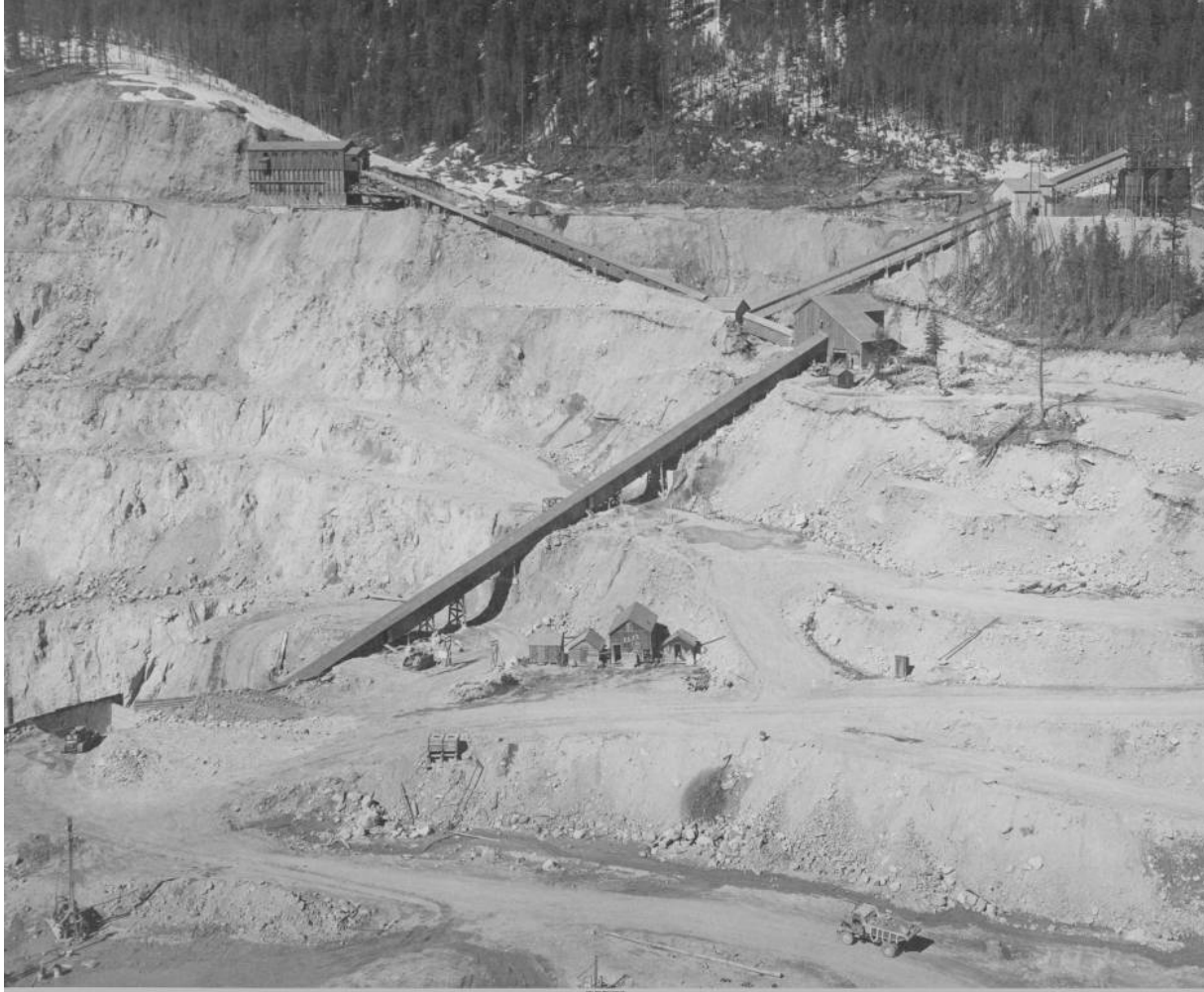
Photo 1: Conveyors and Mill Buildings at Stibnite Mine in 1949 (Source: Idaho State Historical Society, Boise Idaho)
